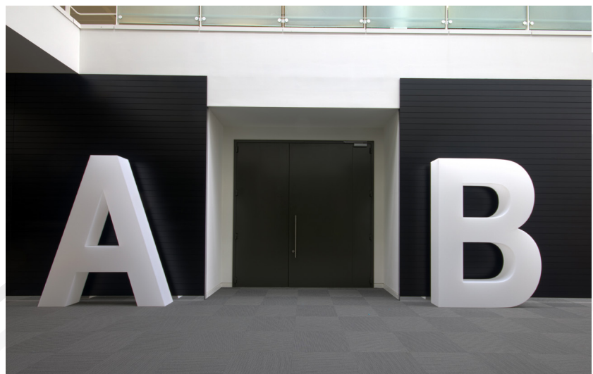
Double acoustic doorset installed at IMG
