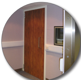
Wood grain paint finishes
